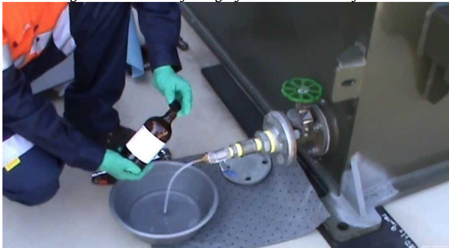
Fig.4.22 Replacing of oil from transformer
