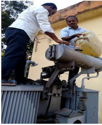
Fig.4.21 Manual filling of oil in the transformer
