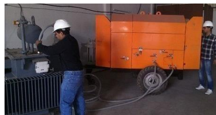
Fig.4.20 Filling of oil in the transformer using oil filling machine
